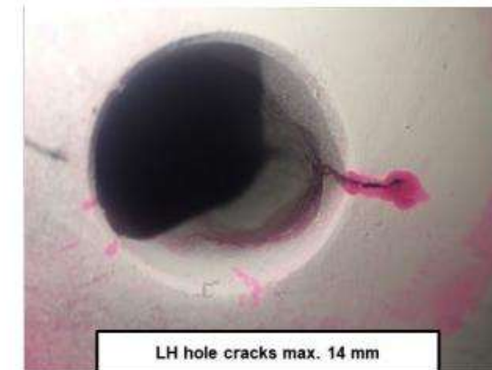
Strain-induced corrosion cracks in main stop valve body
