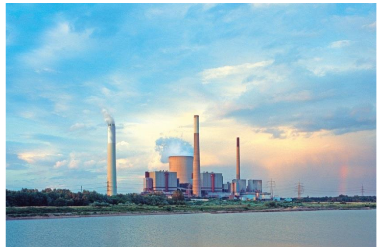
Power plant Voerde. Source: STEAG
