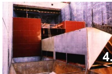
Pic 5 Installation of by-pass dampers
