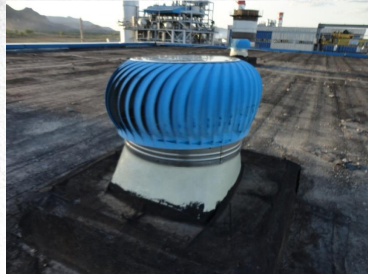
Wind driven Turbo Ventilators
