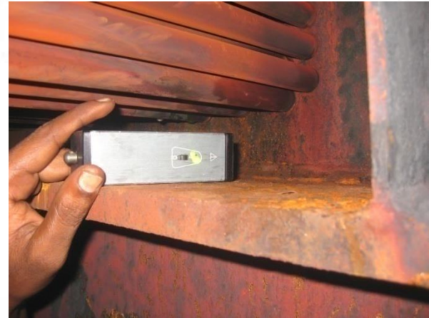
Condenser tube leak test
