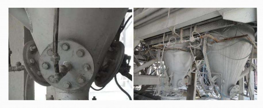
Filling of Buffer Hopper: PE valve not functioning properly, reciprocating design valve provided.
