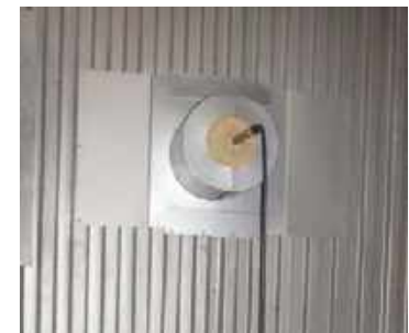
Installation condition of sensor
