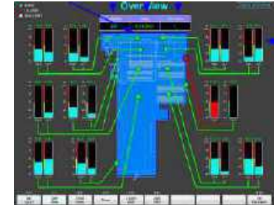
Red part : tube leak detected sensor Screen for indication of tube leak detection
