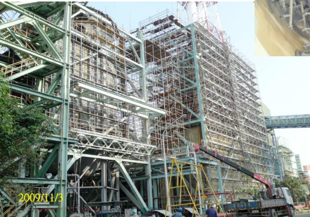
Prescrubber / Cooler Demolition
