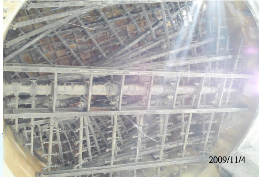
Absorber Slurry Recycle Header Demolition
