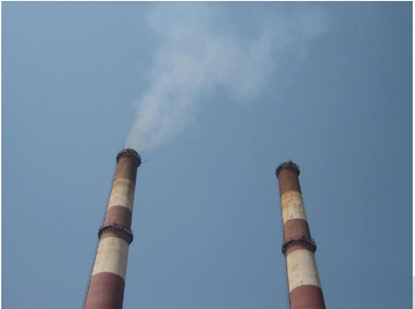
POSCO GWANGYANG #1-4 SINTER PLANT
