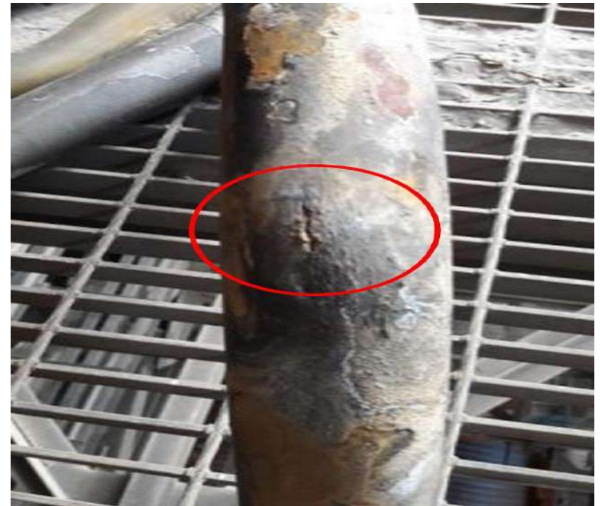
Visual inspection reveals a lot
