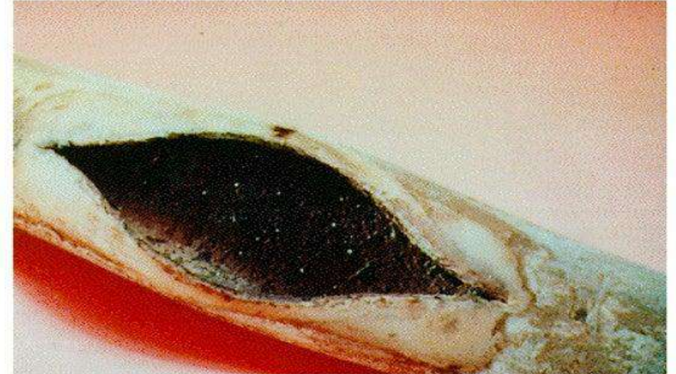
Long Term Overheating
