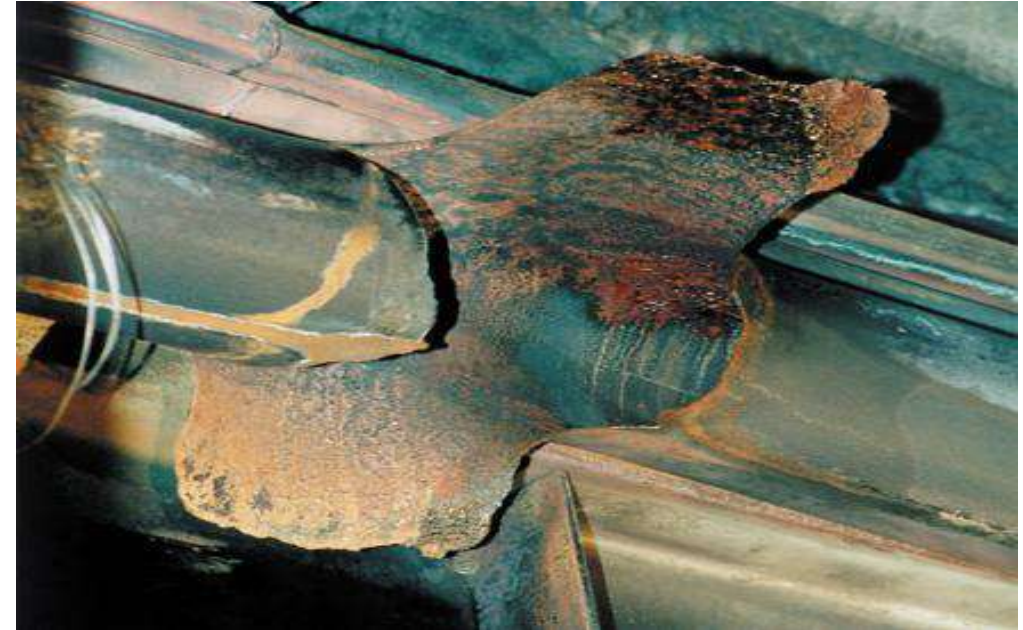
Pictorial view of Boiler tube failure
