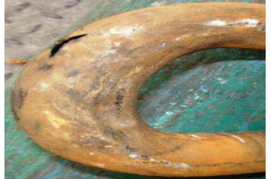
Pictorial view of Boiler tube failure
