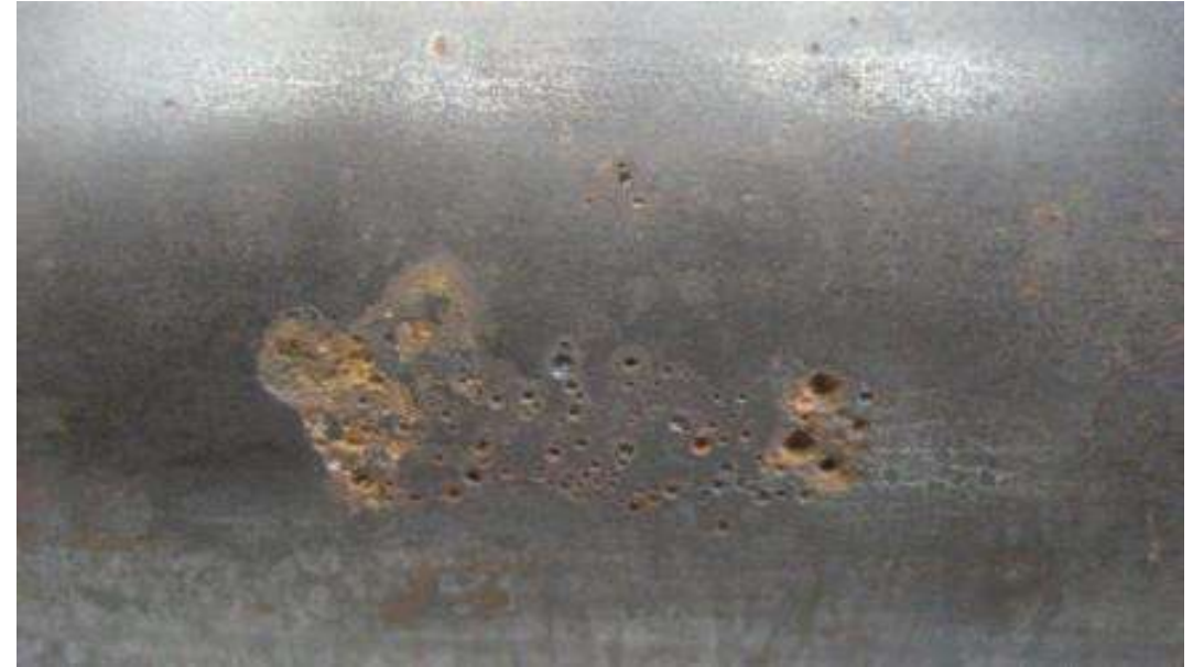
Oxygen pitting failure in Boiler tube
