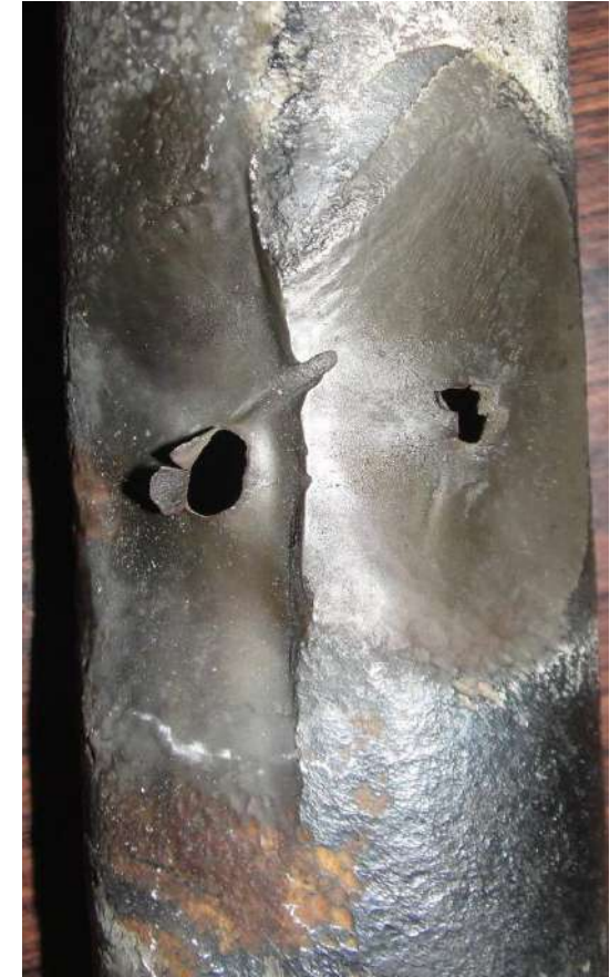
Fly ash erosion in LTSH
