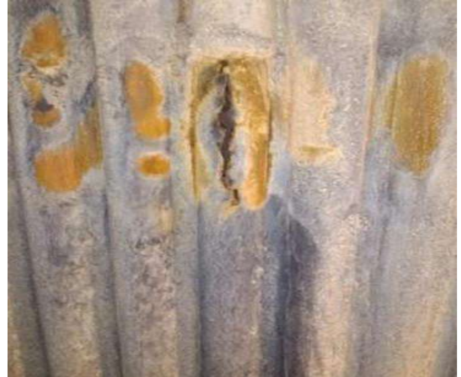
Hydrogen Damage - Thick edged window opening failure
