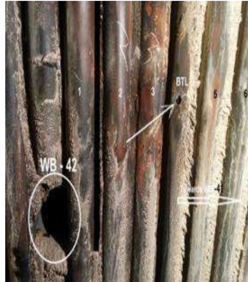
WW erosion due to Soot blower electric control failure
