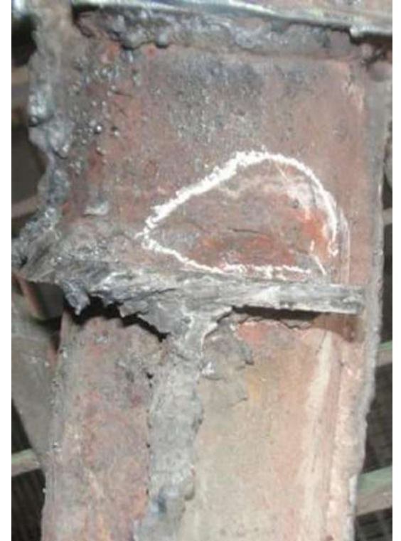
Attachment weld failure in SCW
