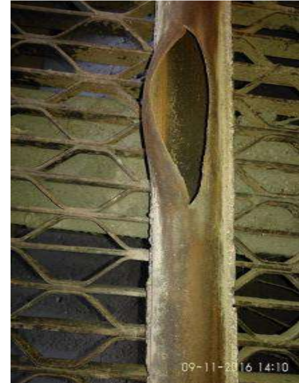
Pictorial view of short term overheating failure
