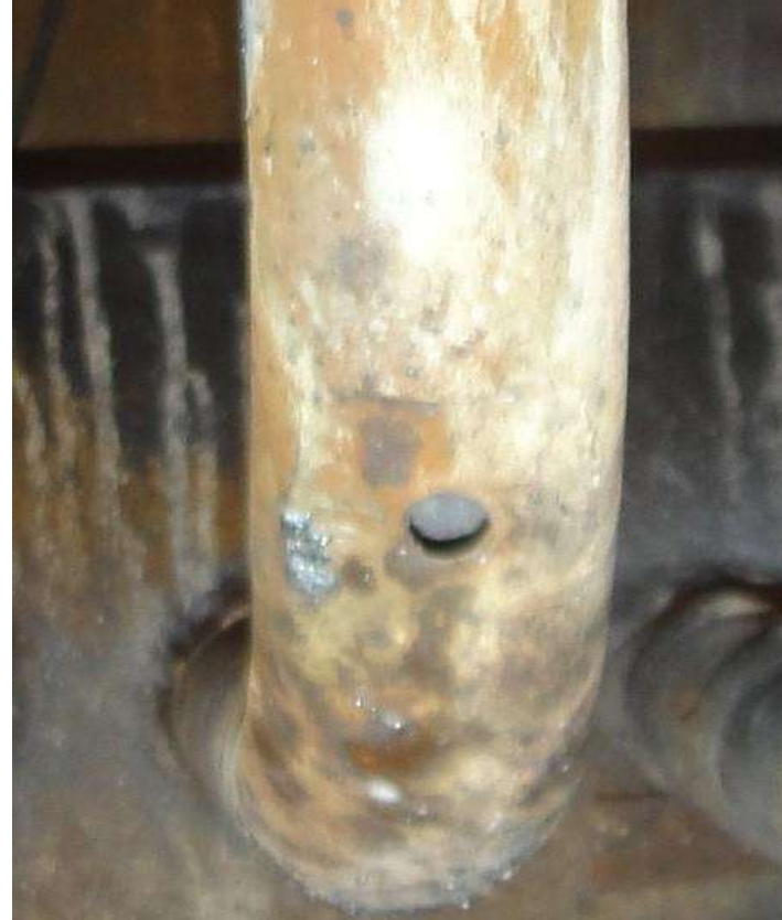
Pictorial view of Boiler tube failure due to erosion
