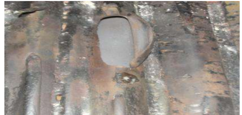
Falling ash erosion in S-Panel
