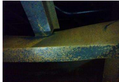
Twisted structural members of condenser
