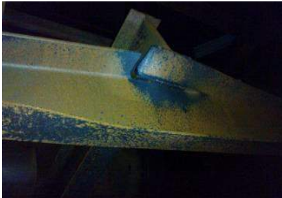
Twisted structural members of condenser
