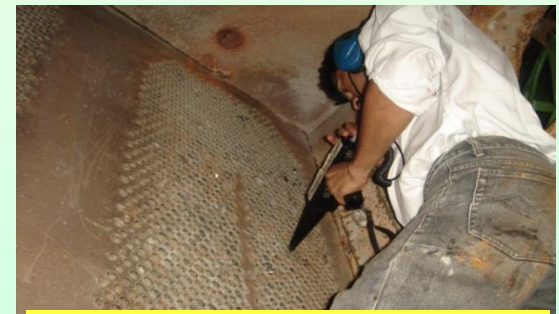
Condenser Tube Leak Detection
