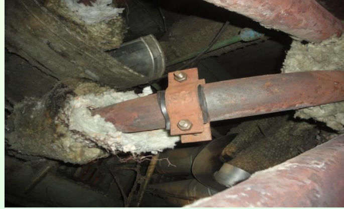
Hole fixed up using clamp
