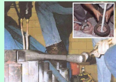
Turbine stud Opening
