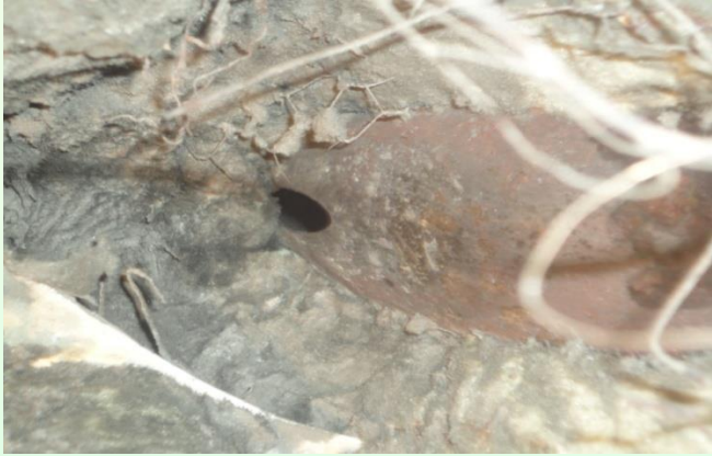
Hole in the CRH strainer drain line
